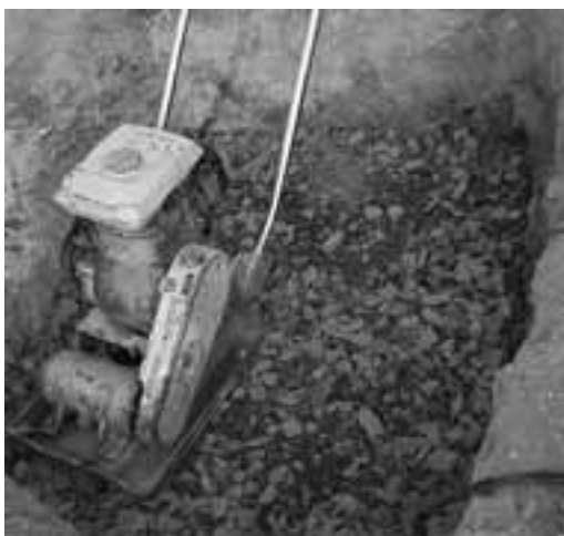
Figure 1 Test pit (gravel)
